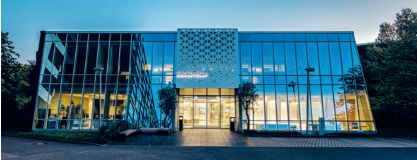
Customer center: TRUMPF impresses customers with its combination of outstanding industrial architecture and superb product quality.
